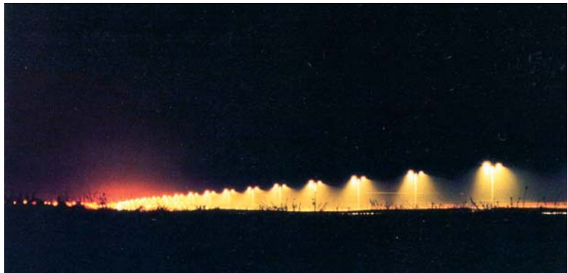
Full Cut Off lights illuminate the road without lighting up the night sky – but notice the sky glow from a settlement in the distance.
