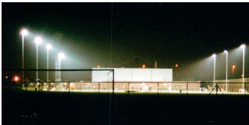
Original (left) and Full Cut Off (right) lighting at a sports ground
