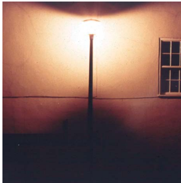
Badly designed lighting spills light horizontally and upwards
