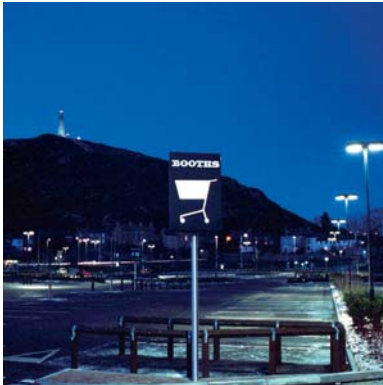
Good example of outdoor lighting in large retailers car park, Ulverston
